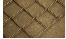
On top of the weldmesh, the group laid sand, cement and gravel, which they mixed with their spades. The next job was to carry water
